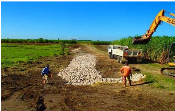
Works on the access road and diversion bank. Photo: QDAFF
