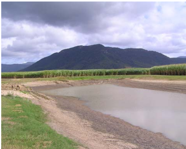
Detention basin acting as both a sediment trap and a sump for a larger ring tank. Photo: QDAFF
