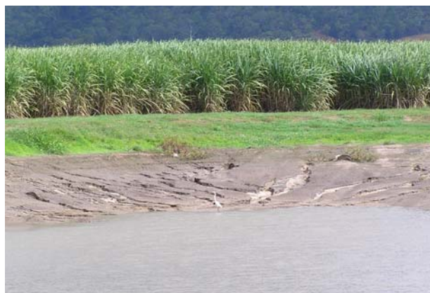
Detention basin and grassed headland showing sediment being trapped from recent flow event. Photo: QDAFF
