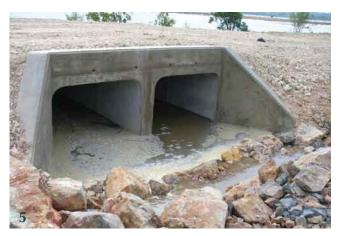
Photo 5: New culvert through roadway barrier now connects freshwater wetland to brackish water (photo: Rockhampton Regional
