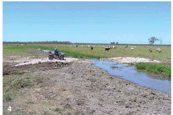
Photo 4: Rock erosion control structure installed in outlet channel of Horseshoe Lagoon (photo: Jim Tait)
