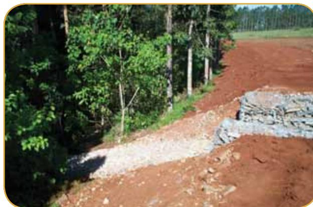
*Example of a rock gabion 'leakage' weir outlet from a sediment trap that discharges flows direct to a creek. Note the rock ramp (chute) that prevents bank erosion and the formation of gully heads when the trap is overflowing. (Photo by Joe Rhodes).*
