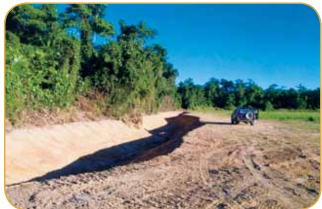
Example of detention basin/sediment trap. Note the steep batters, which required less production land. (Photo by Joe Rhodes).
