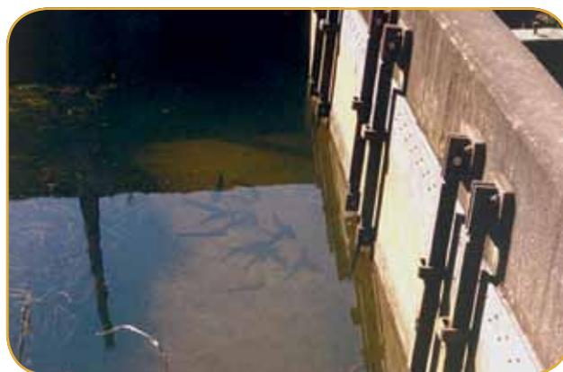
This floodgate on the upper end of a tidal system prevents the inflow of tidal water and fish. Note the fish blocked at the floodgate. (Photo by Matt Gordos).
