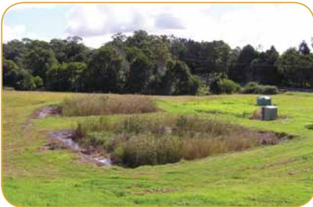
A reed bed wetland treatment system at a production nursery in New South Wales. This system, which captures and treats site runoff and irrigation water, has saved the nursery 124,000 litres/day. (Photo by Ian Layden).
