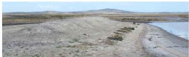
Bank blocking channel flow from right to left, with bypass.
