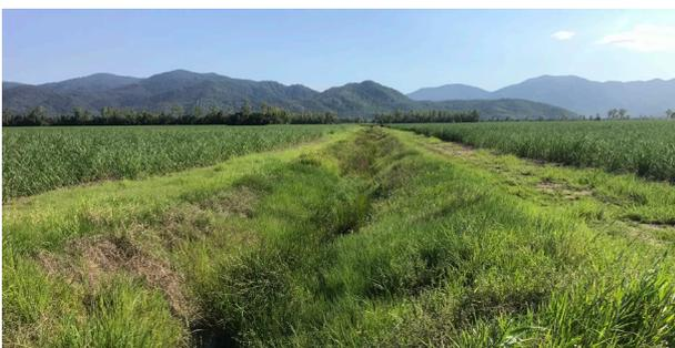
Figure 1 Vegetated drains can reduce nitrogen through wetland processes. Queensland Government
