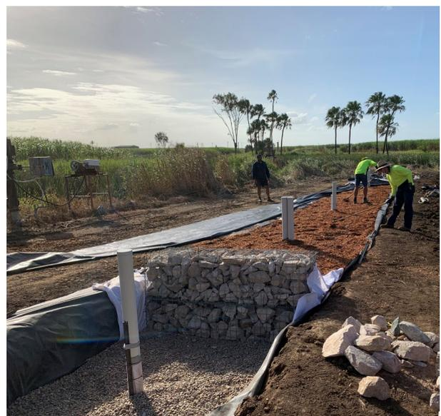
Figure 2 This woodchip bioreactor bed was effective at removing DIN from irrigation tailwater from a cane farm. Queensland Government
