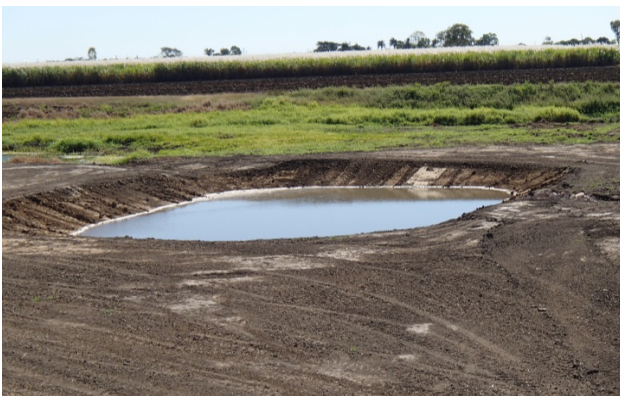
Newly constructed sediment basin. Photo: QDAFF
