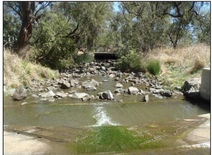
**Figure 11** Fish passage structures on Bowenville Gauging Station Weir, Oakey Creek, Queensland including rock ramp and baffles (Source: Andrea Prior).
