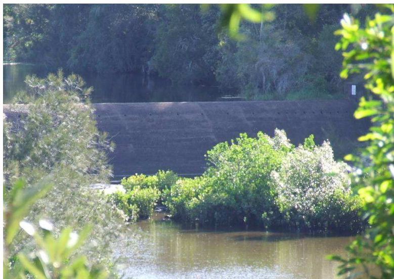
Burrum River Barrage 1 does not have an effective fishway and blocks connectivity to the freshwater reaches of the river system
