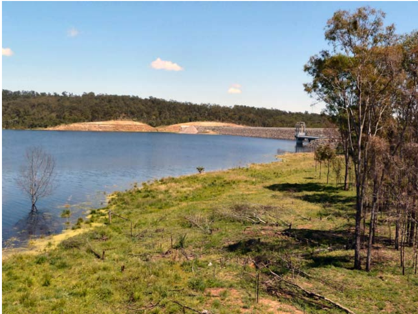
Photo 1: Bjelke Petersen Dam. Photo: Steven Howell, DERM
